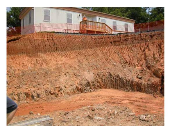
Due to the difference in site grading between the school level and the field level, there would be significant site excavation for a new addition should it be at the same floor level as the school. The site is known to contain some ledge which will have a cost impact on the construction.
